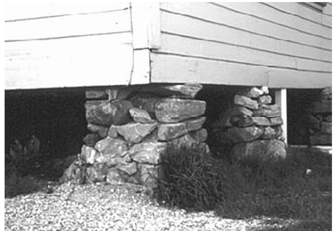
Figure 16 - This is an unreinforced stone foundation. They typically fail during earthquakes.
